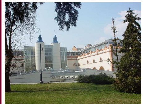
Veszprem of Hungary: County Library Building
